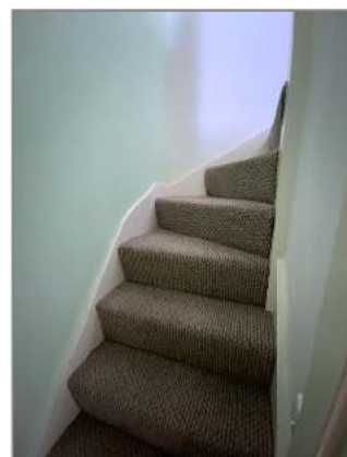
Photo - 102 No handrail to second floor stairs
