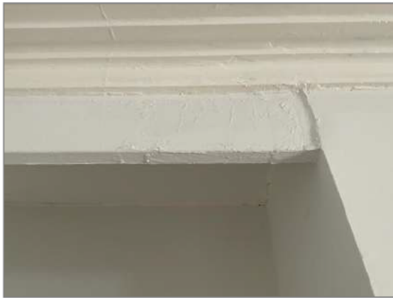
Photo - 56 Poor finish to timber infills either side of living room chimney breast
