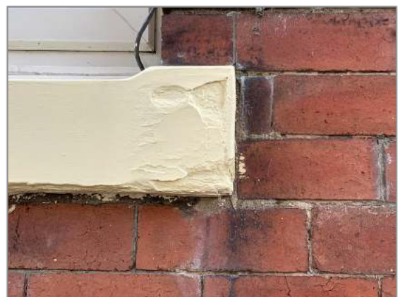
Photo - 20 Spalled stone to lintels and sills
