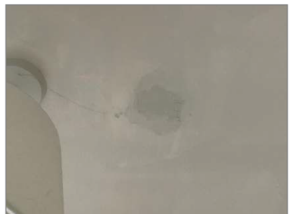
Photo - 40 Patch repair to landing ceiling
