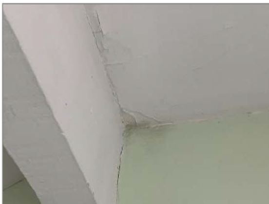
Photo - 45 Possible damp staining above second floor stairs
