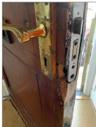
Photo - 31 Impact damage to front door
