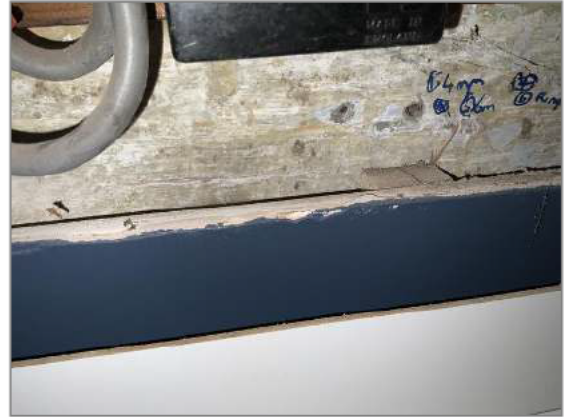
Photo - 51 No damp proofing visible around edges of dry lining to kitchen
