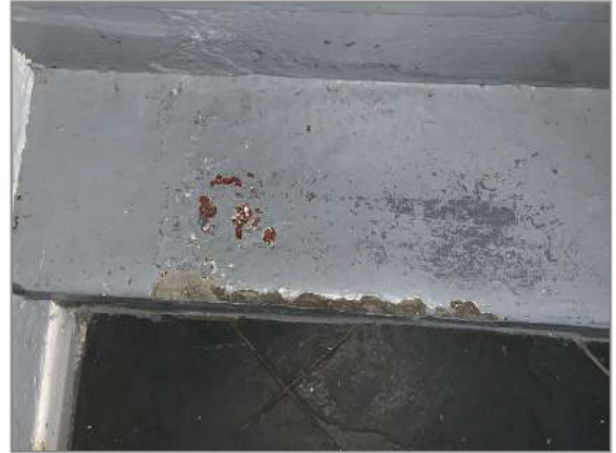
Photo - 71 Peeling paint to kitchen steps
