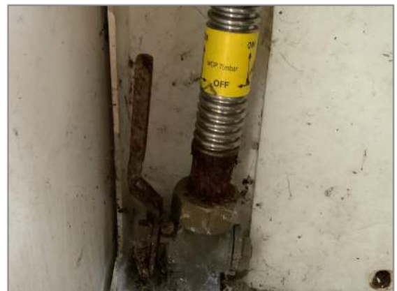
Photo - 108 Corroded pipe
