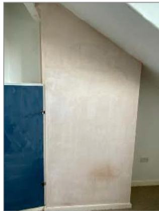
Photo - 64 Recent re-plastering to second floor bedroom chimney breast
