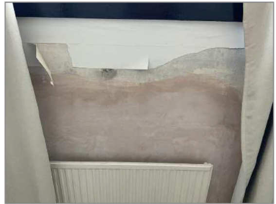
Photo - 63 Peeling wallpaper and patch repairs to plaster to second floor bedroom wall
