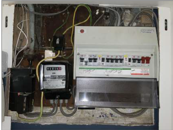
Photo - 106 Electric meter and consumer unit
