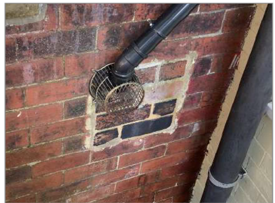
Photo - 18 Bricked up alteration
