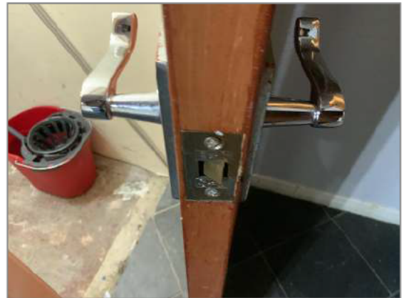
Photo - 98 Broken latch mechanism to lower ground floor cupboard door
