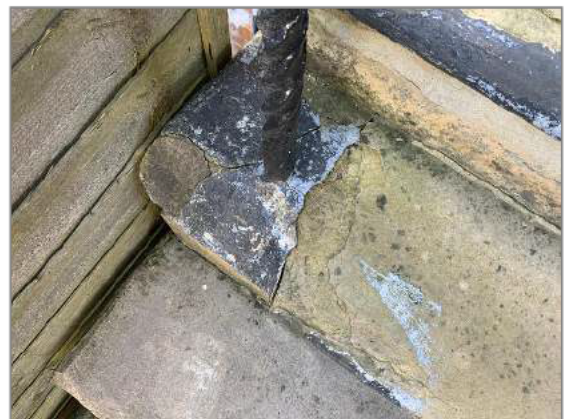
Photo - 126 Cracked stone step and handrail loose
