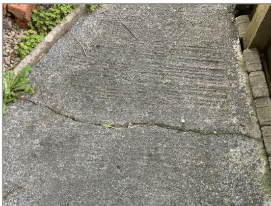
Photo - 119 Crack to concrete path
