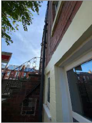
Photo - 114 PVC soil and vent pipe
