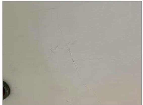
Photo - 44 Fine cracks to second floor bedroom ceiling
