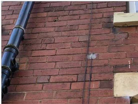
Photo - 23 Open mortar joints
