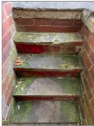
Photo - 115 Cracked stone treads to steps to lower ground floor
