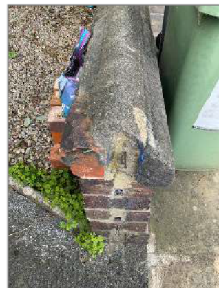
Photo - 120 Damage and movement to front boundary wall
