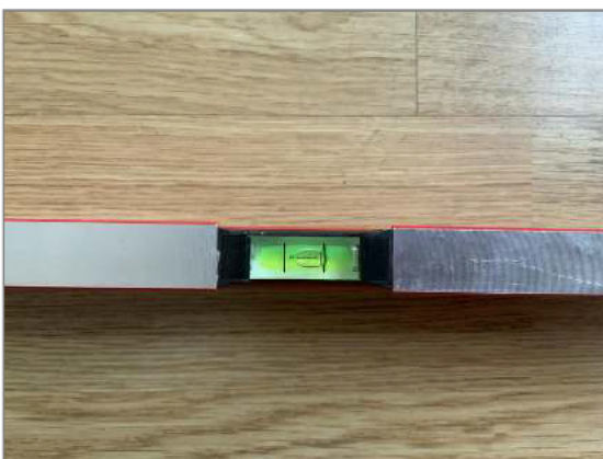
Photo - 74 Living room floor slopes approximately 2cm front to back
