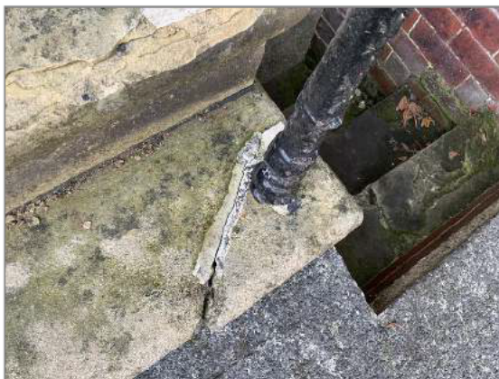
Photo - 125 Cracked stone step
