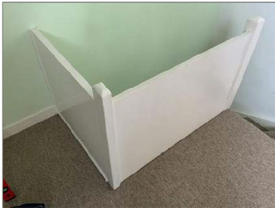
Photo - 103 Second floor landing guarding too low at approximately 700mm
