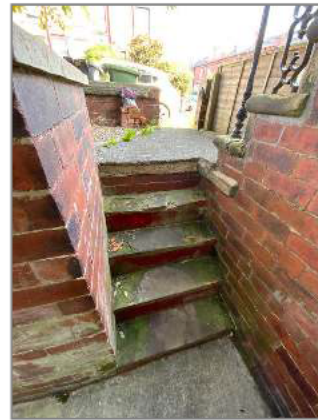
Photo - 116 No handrail to lower ground floor steps
