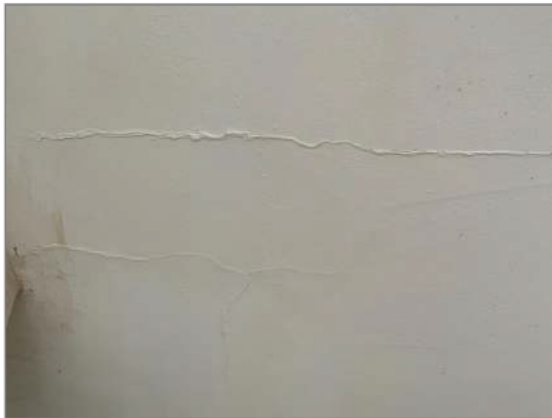
Photo - 47 Cracks to second floor bedroom ceiling
