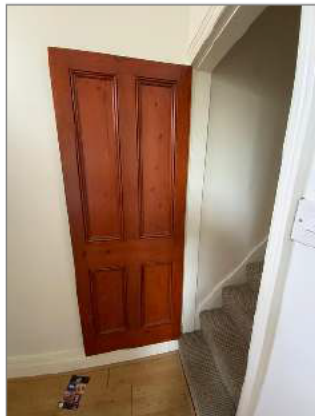
Photo - 99 No fire doors fitted
