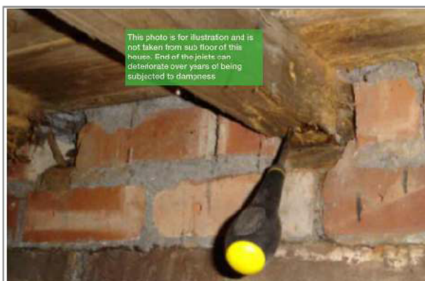
Photo - 86 Not of this property - show to highlight the effects of damp/rot to subfloor timbers
