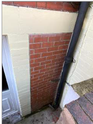
Photo - 15 Bricked up door opening to lower ground floor
