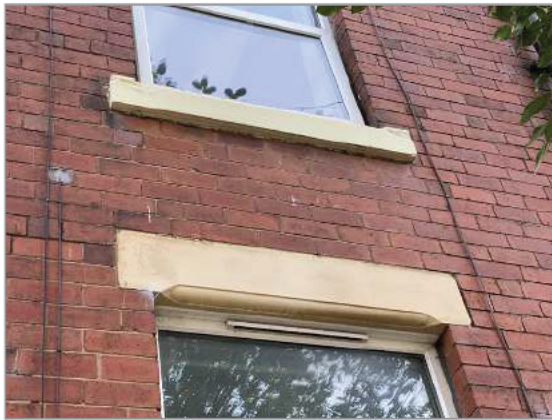
Photo - 21 Stone lintels and sills
