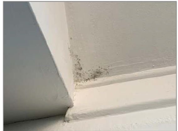
Photo - 48 Black mould growth to dormer ceiling
