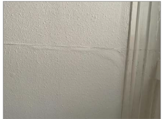
Photo - 38 Peeling wallpaper to living room ceiling
