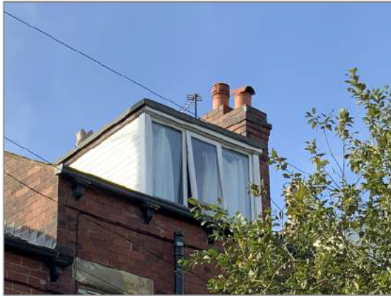
Photo - 25 Staining to dormer windows
