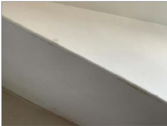
Photo - 49 Staining may indicate leak between main roof and dormer
