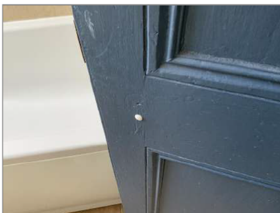
Photo - 101 No external handle to bathroom door
