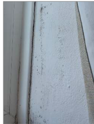
Photo - 65 Black mould growth around second floor window opening
