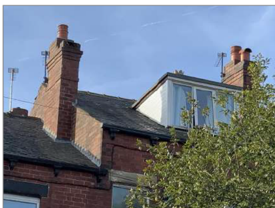
Photo - 6 Main roof covering and flat roof to dormer
