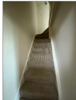
Photo - 100 No handrail to first floor stairs
