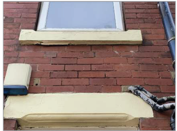
Photo - 22 Open mortar joints
