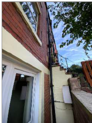
Photo - 112 Cast iron soil and vent pipe
