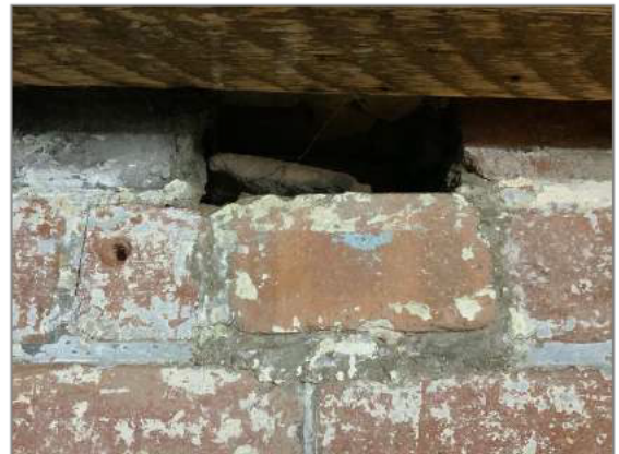
Photo - 53 Missing brick from kitchen wall
