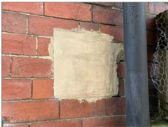
Photo - 17 Rough patch repair
