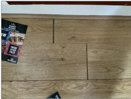
Photo - 76 Loose laminate to living room floor
