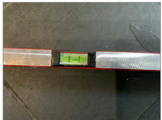
Photo - 69 Lower ground floor slopes significantly
