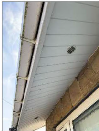
Photo - 56 Some ventilation is provided to eaves at soffits
