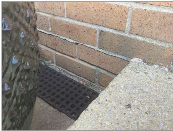
Photo - 23 Rear elevation damp proof course is level with internal finish floor level
