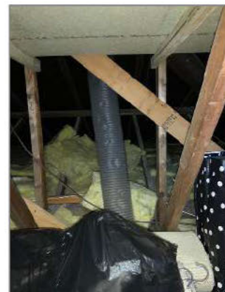
Photo - 69 Bathroom extraction ducting to roof is dented throughout its length
