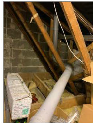
Photo - 138 Soil vent pipe has been relocated from its original exit in roof.
