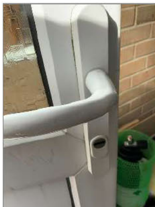
Photo - 40 Rear door to conservatory has a secure by design handle protecting cylinder
