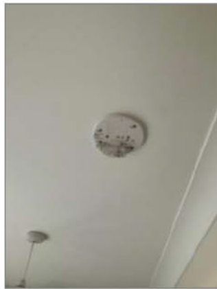
Photo - 156 Utility smoke alarm required a new battery
