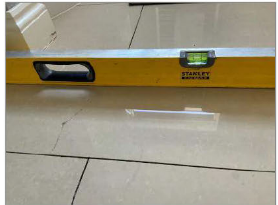
Photo - 95 Bathroom floor drops to rear by approximately 3mm/m
