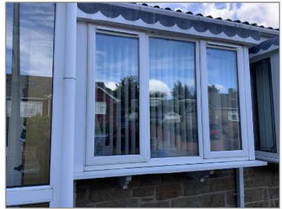
Photo - 28 Kitchen bow window is supported by timber noggins set into masonry behind and below
