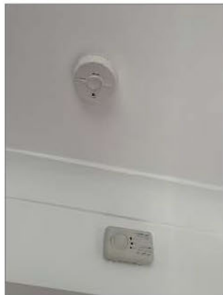
Photo - 158 Living room has a carbon monoxide detector and battery smoke alarm
