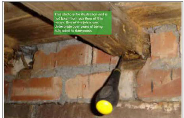
Photo - 99 Not of this property - show to highlight the effects of damp/rot to subfloor timbers
