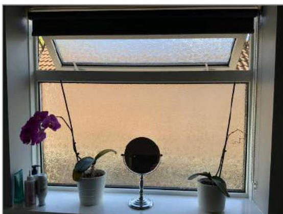
Photo - 35 Bathroom window hinge to front has become sprained preventing window closing fully at top.
