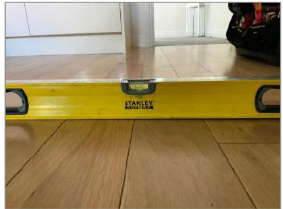
Photo - 89 Kitchen floor drops to left and rigging center
