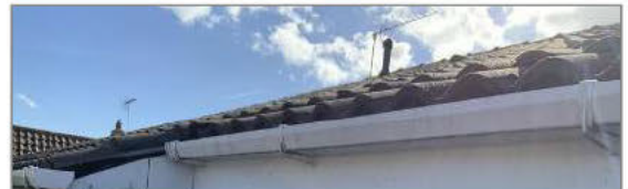
Photo - 7 Verge pointing is reasonably secure, mortar has shrunk slightly as it dried out
