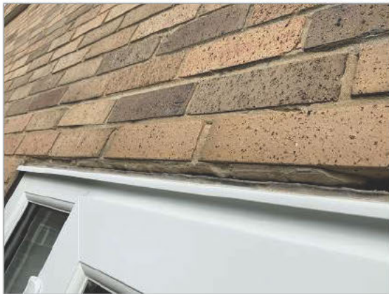
Photo - 25 Pointing to rear French doors and steel lintel
